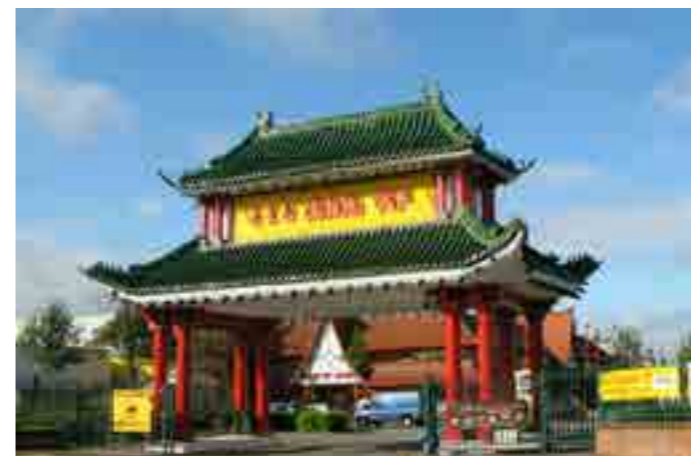
5. Wing Yip supermarket, wholesaler and distribution centre.
