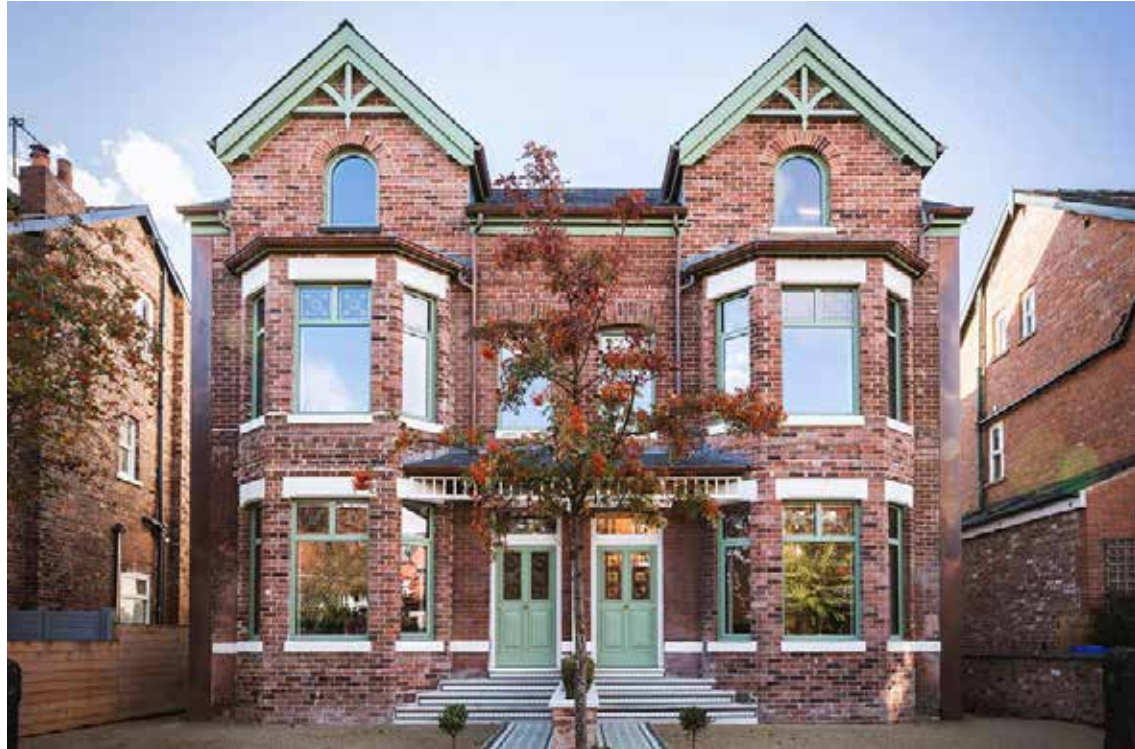
Passivhaus retrofit by Ecospheric
