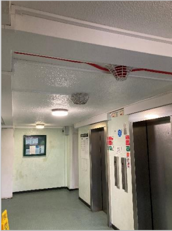
Photo 3 Typical lift lobby entrance hall
