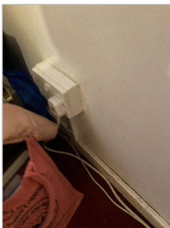
Photo 23 Surface mounted trunking to sockets added
