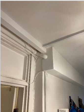
Photo 41 Retrofit sprinkler installation
