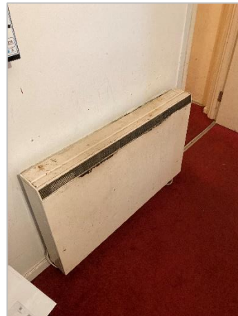
Photo 22 Typical storage heater
