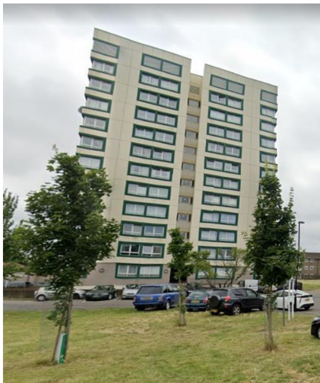
Fig 1 View of South elevation of 58-108A
