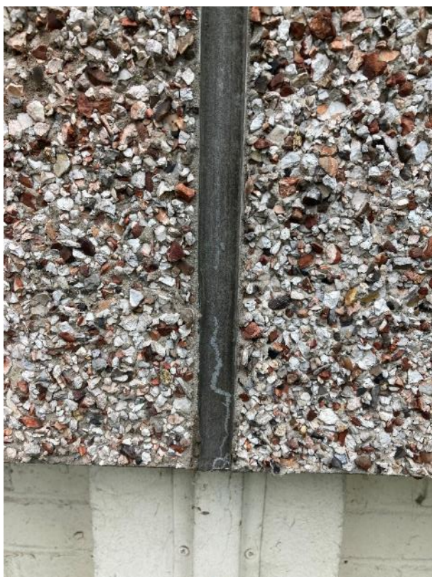
Fig 9 Close up of vertical joint between panels
