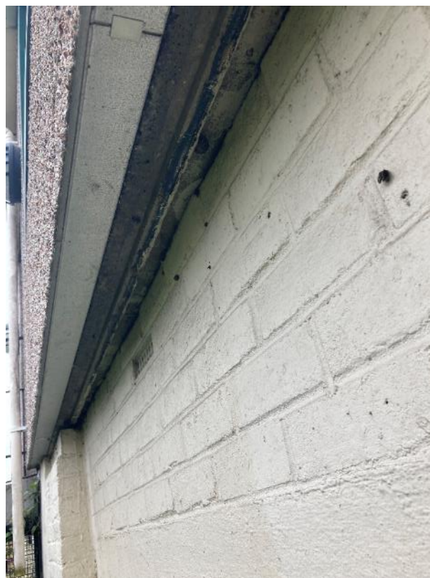
Fig 10 Underside of rendered concrete panel at ground floor level
