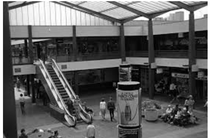
↑ In the 1990s, the centre was almost completely rebuilt to an atrium design © Neil Clifton
