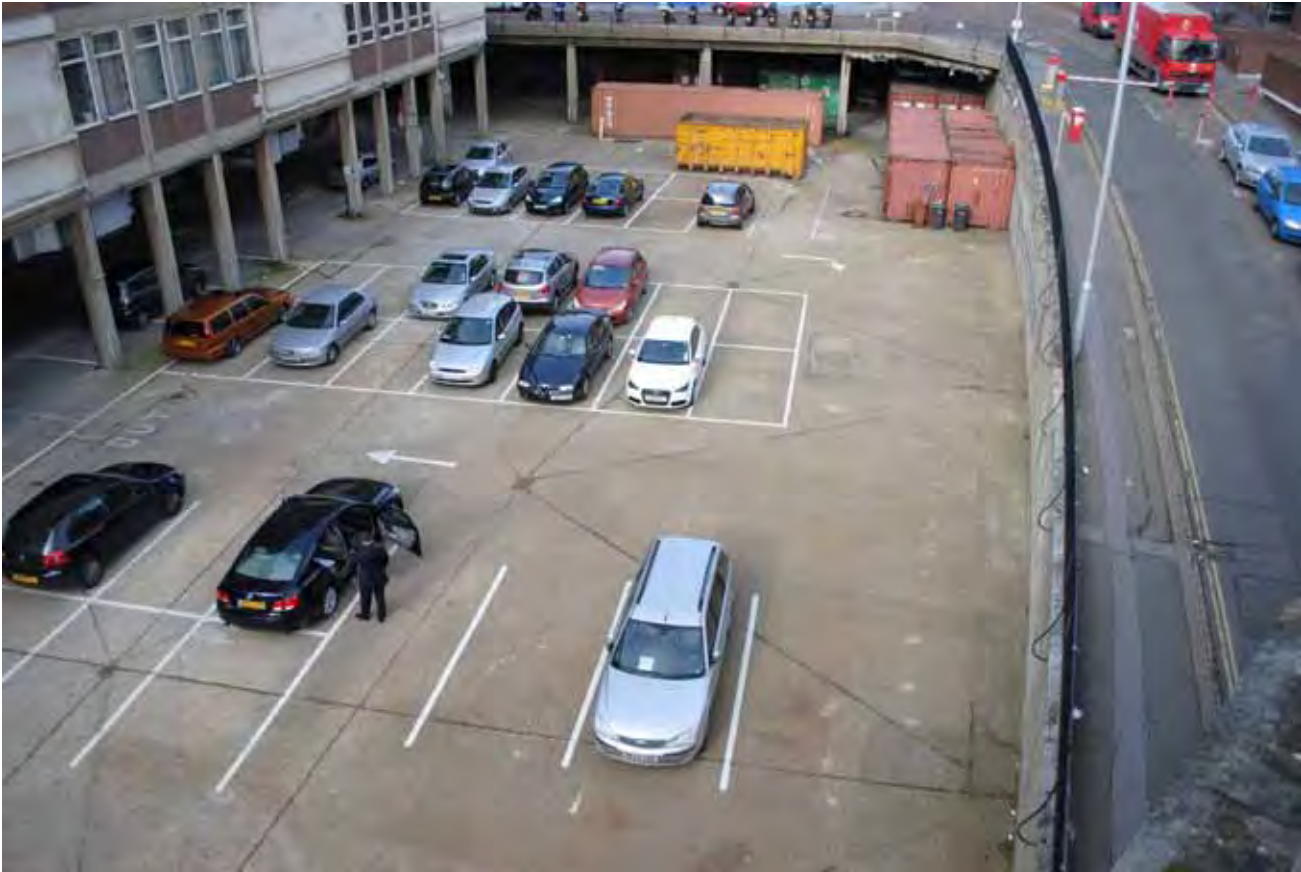
Figure 8.2 Croydon College underground car park
