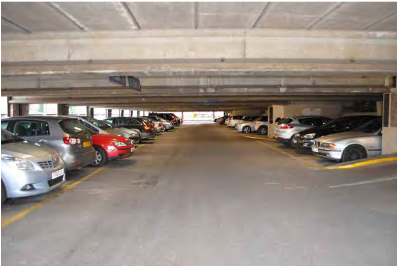
Figure 8.1 Fairfield multi-storey car park
