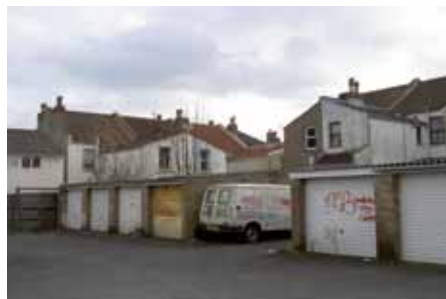
Although this space is overlooked, it is physically isolated from the houses. By the time residents can reach the garages, any vandals will have gone.
