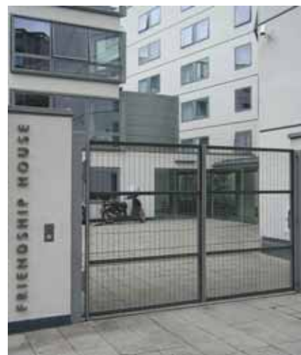
In this UK example, the security of the development has been reinforced by restricting access into the grounds. This should be a last resort as it increases the fear of crime by suggesting the area is unsafe.
