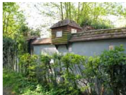
Planting to protect a blank wall.
