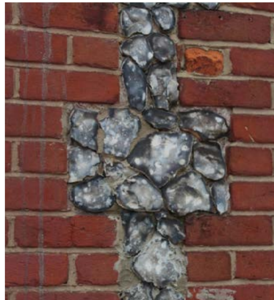
132. Knapped flint and red brick used on Nos. 1-3 (locally listed) on Coventry Road
