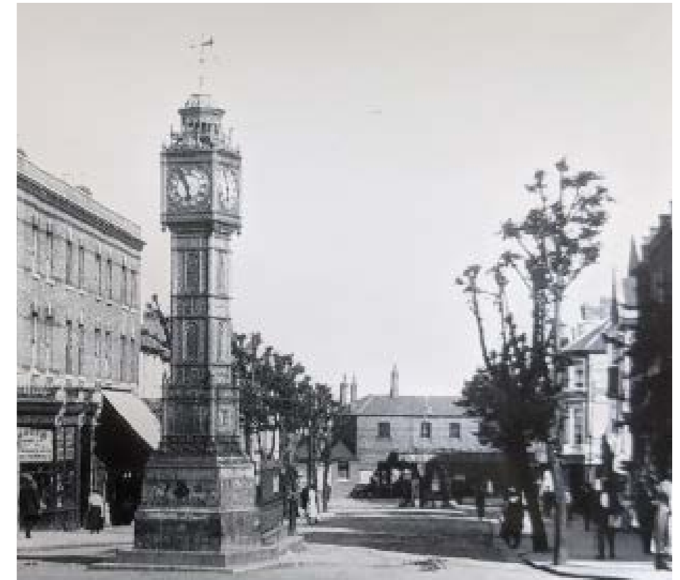
33. Clock Tower (source: Croydon Archives PH/96/4161)
