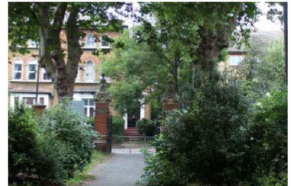
59. View north towards brick piers on Selhurst Road, originally located on Olivers Grove, now adjacent to the Holy Innocents Church
