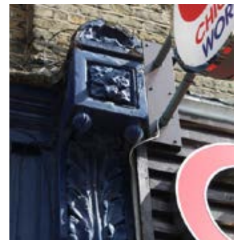
83.Historic shopfront detail
