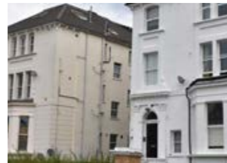
91. Painted render with sash windows
