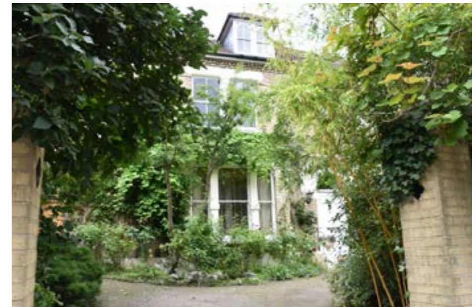
114. No. 76 Warminster Road, demonstrating the leafy character and grand architecture of the area
