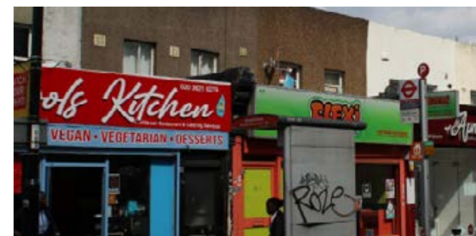
137. Example of modern shopfronts and advertisements, which detract from the historic character of the area
