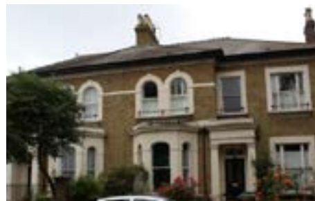
86. London stock brick, stucco, and slate roofing
