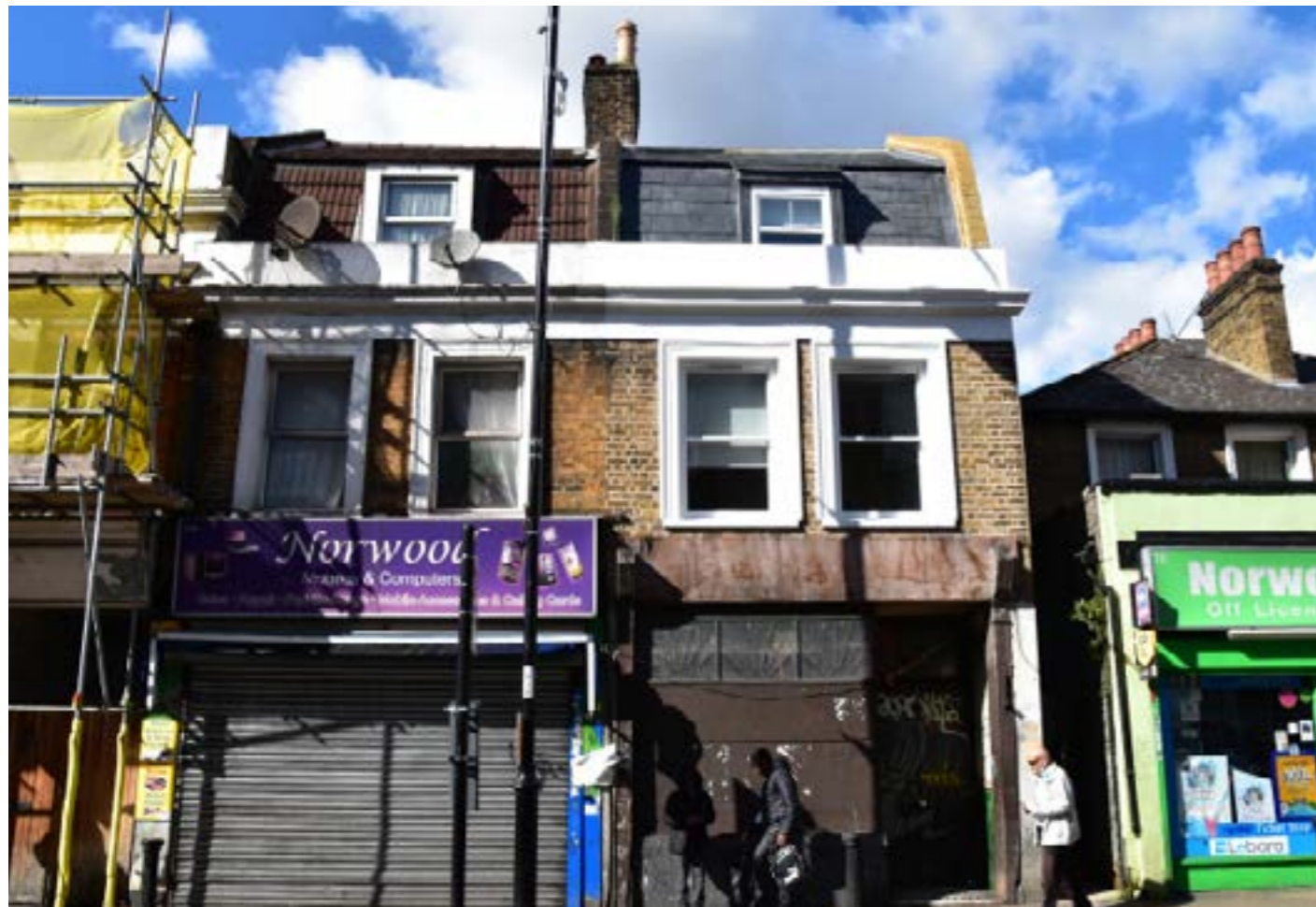
80. Kennedy's Sausages, Grade II Listed, currently on the Heritage at Risk Register
