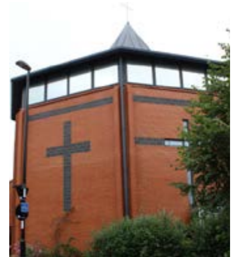
123. South Norwood Baptist Church, Holmesdale Road
