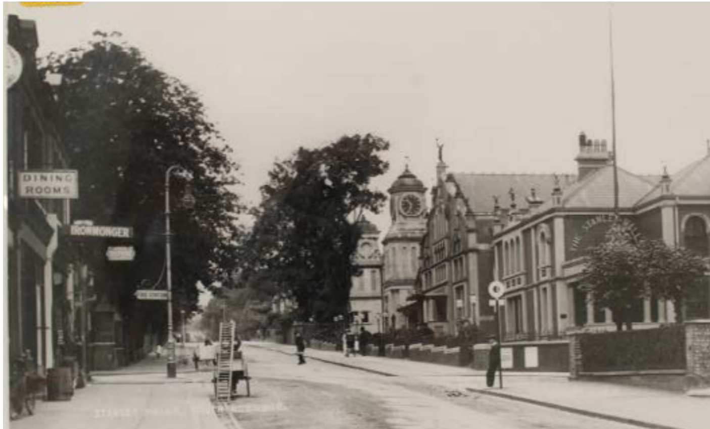
34. Stanley Halls South Norwood Hill (source: Croydon Archives 142.4)
