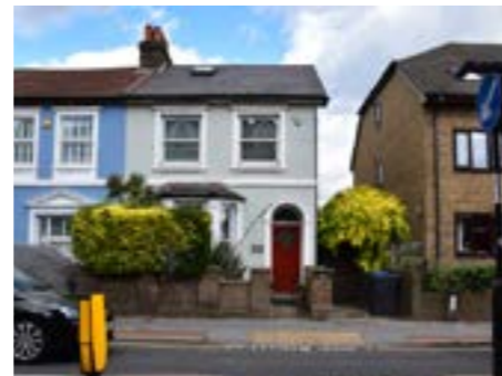
57. Brick boundary on Portland Road, with iron gate and hedge
