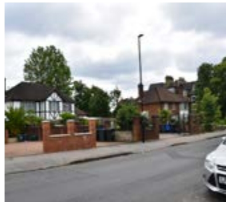
117. Twentieth century development, within large plots which are characteristic of the area
