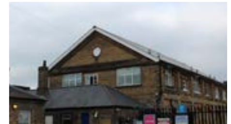
8. The goods shed at Norwood Junction Station
