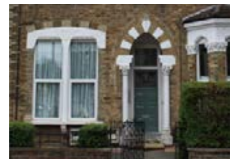
84.Decorated door and window surrounds, and arched opening and stone dressings. Ironwork railings and gate still in place.
