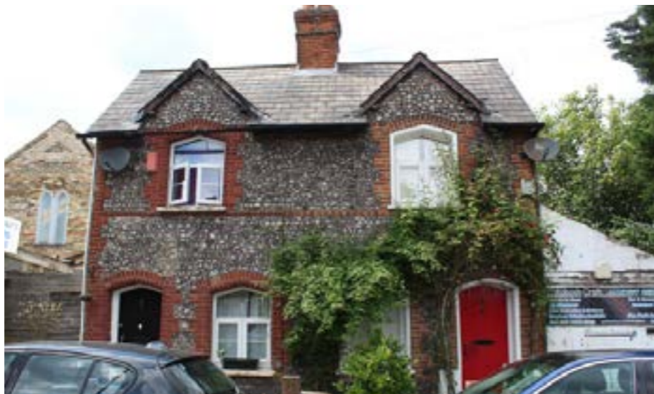
63. Victorian flint cottages on Coventry Road (Locally Listed)
