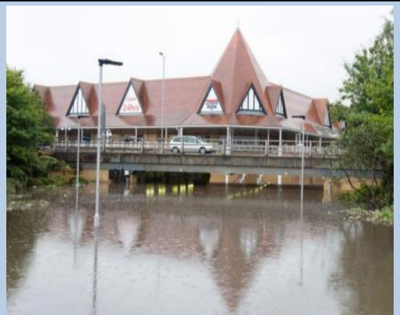
Figure 1: Purley Cross underpass (Croydon, 2015)
