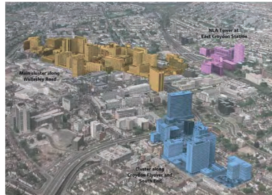
Fig 8 Existing tall building clusters in 2013 (from Croydon OAPF)
