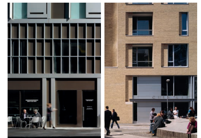
Fig 253 The base: Welcoming, attractive and clearly defined entrances which relate positively to the surrounding street
