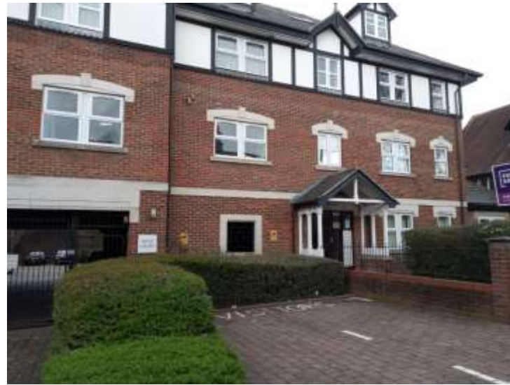
Purpose built block of flats with well kept purpose built bin store
