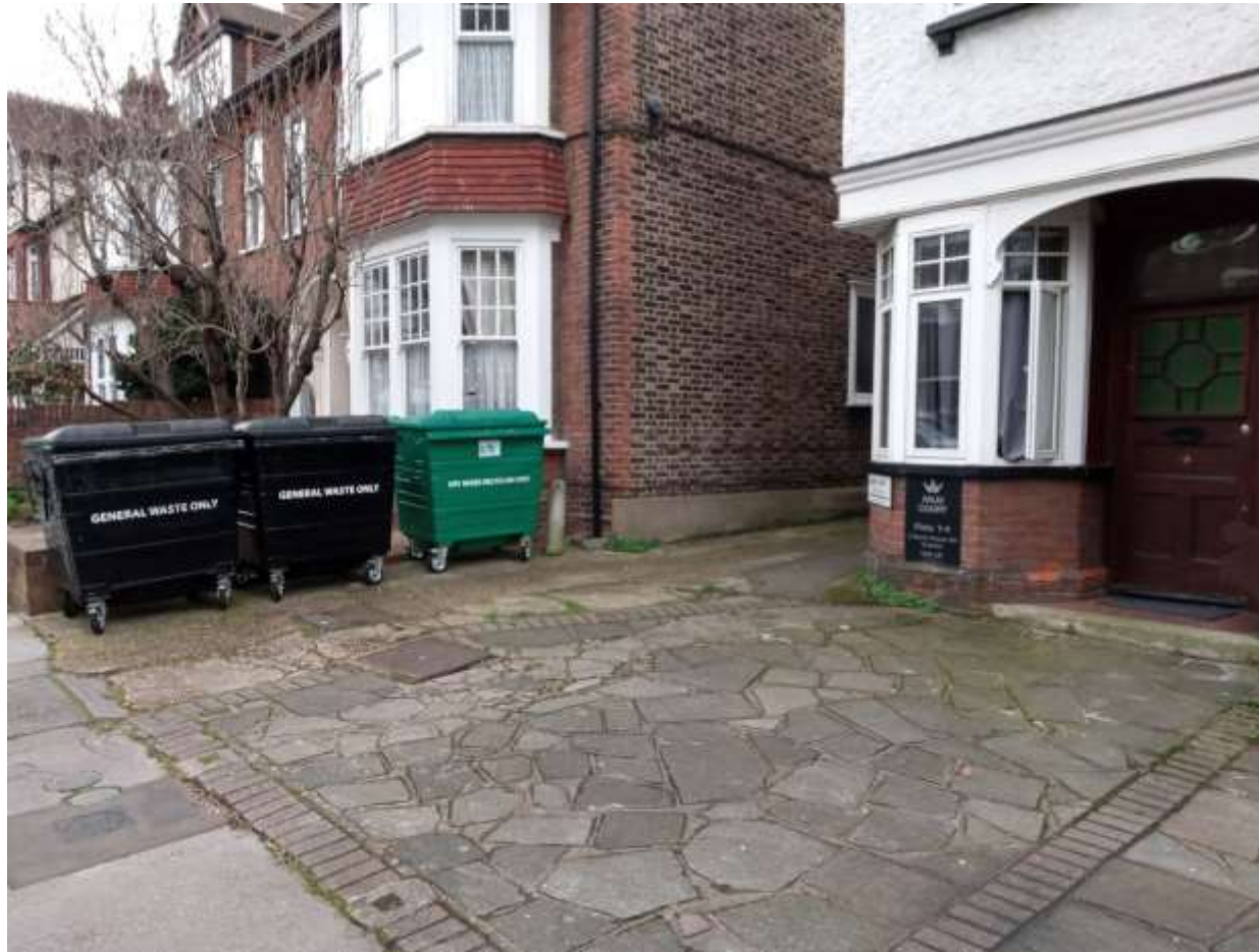
House conversion of six flats with well presented hire bins
