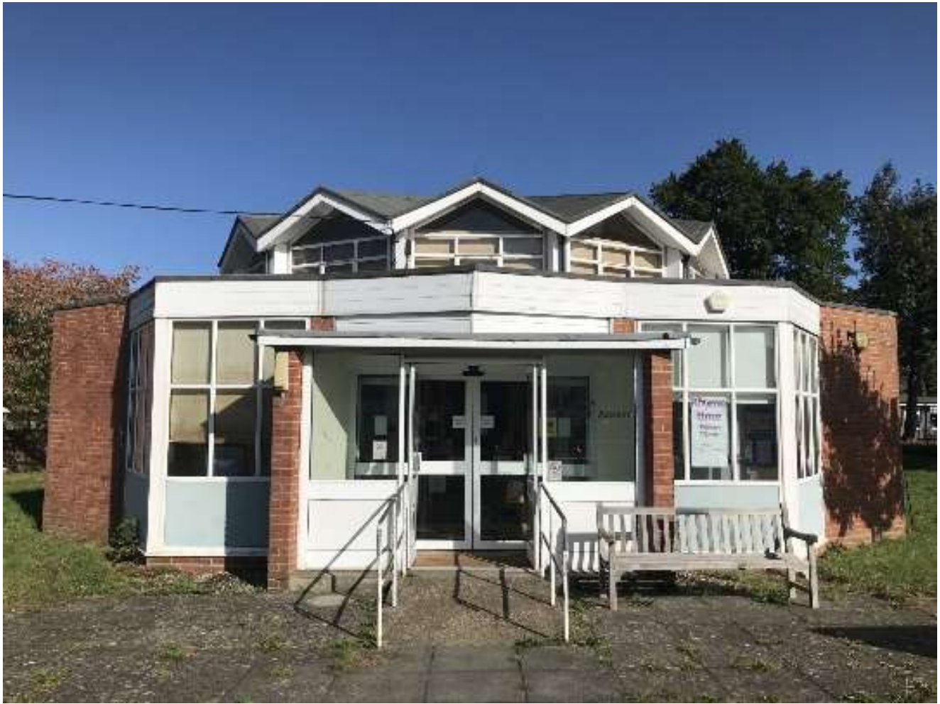
Bradmore Green Library Building, Bradmore Way, Coulson, CR5 1PE
