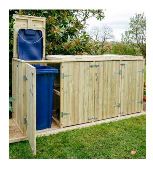
This bin store is not suitable due to the low lintel and chain attached to bin, which will prevent collection.
