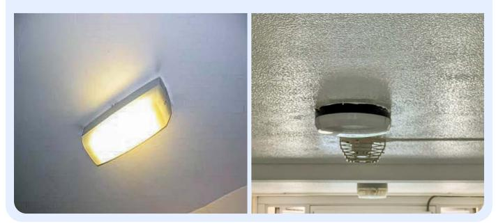
The light shade is in poor condition and there is evidence of old cobwebs and very dirty casings and surface.
