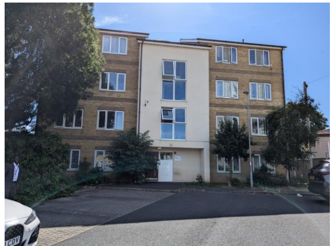
Figure 5: Façade of 110a Regina Road
