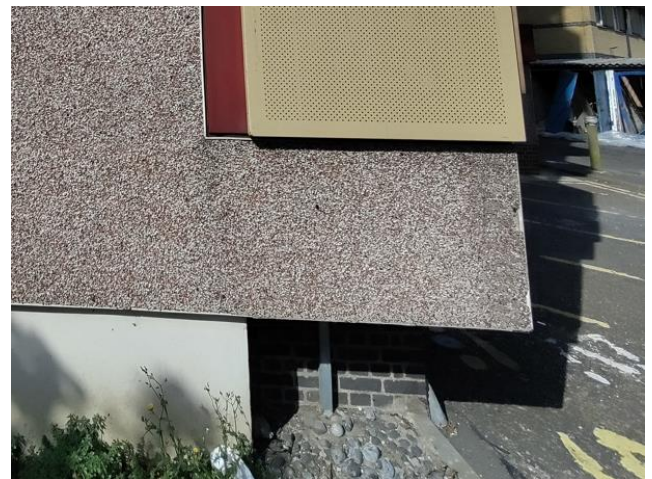
Figure 14: External brick on the facade
