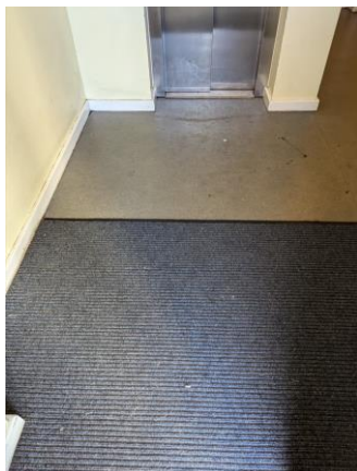
Entranceway to building
