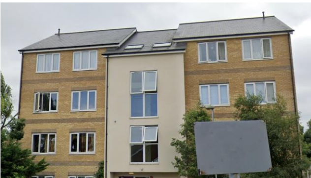
Figure 21: North facing façade showing the pitched roof
