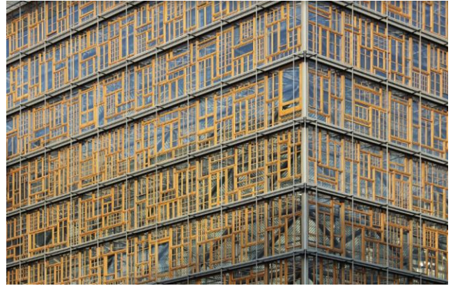
Figure 33 EU Headquarters famously incorporates a patchwork of 3,750 recycled wooden window frames procured from renovation or demolition sites across Europe in its façade. – Image: Dezeen
