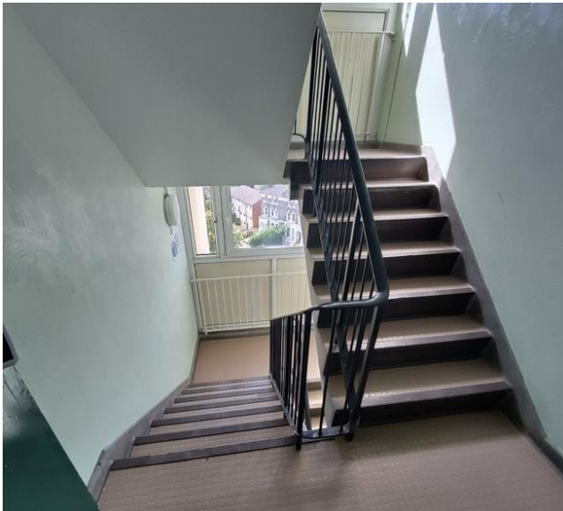
Figure 17: Timber staircase for the Annexe
