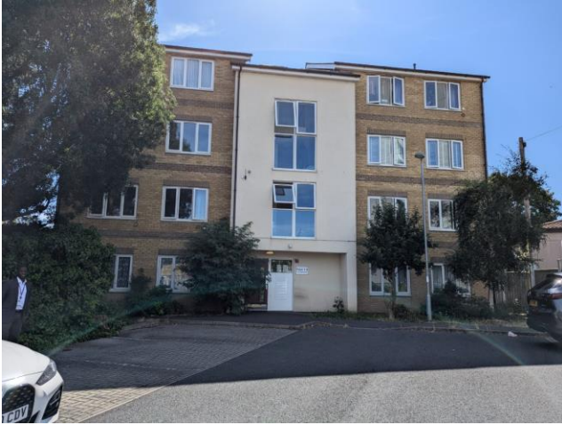
Figure 20: PVC windows on the facade
