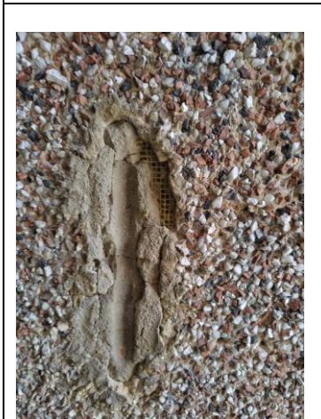
External façade to ground floor showing concrete system
