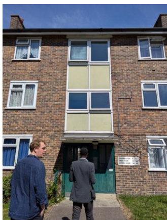
Façade from Sunny Bank
