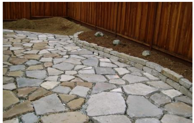
Figure 29: Reusing broken up concrete within landscaping, paving and kerbs is a good way to promote direct reuse onsite – Image: https://www.terranovalandscaping.com/90/
