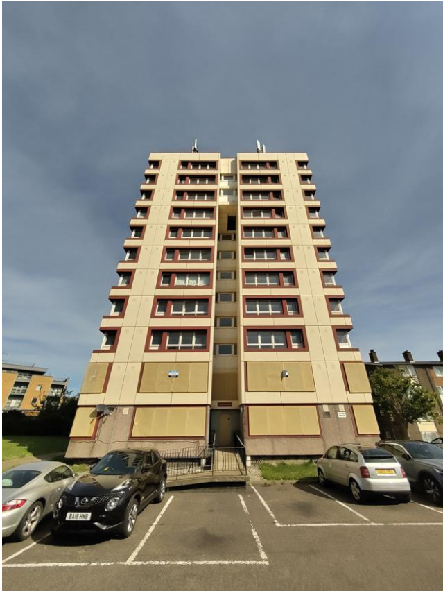
Figure 3: Façade of 1-87 Regina Road
