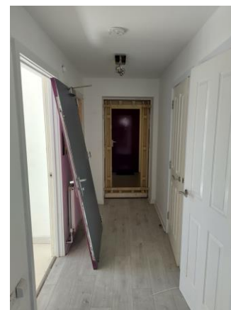
Hallway within flat
