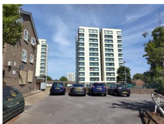
South façade view from Sunny Lane
