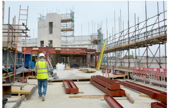
Figure 31: Reclaimed steel used at Holbein gardens, HTS 1
