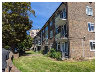
Façade from Sunny Bank
