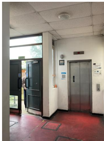
Hallway to lift and fire exit
