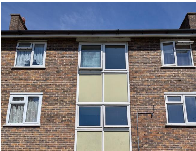
Figure 25: Southwest façade showing brickwork and windows
