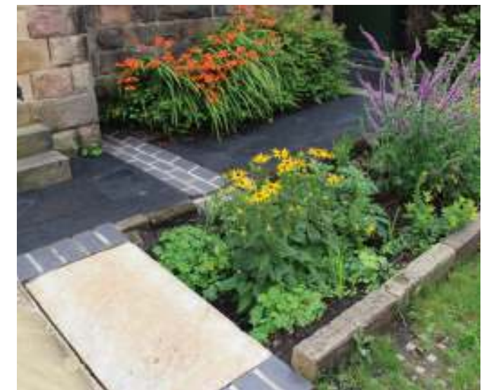
Strutts Centre, Belper. Brick channels collect roofwater for linear raingarden with garden style planting.
