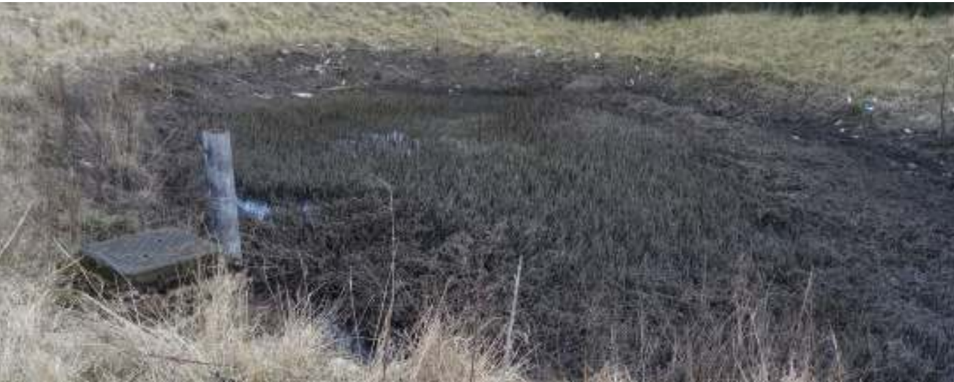
A basin without source control can result in silt, oil and litter pollution that reduces both the amenity and biodiversity value of the feature.
