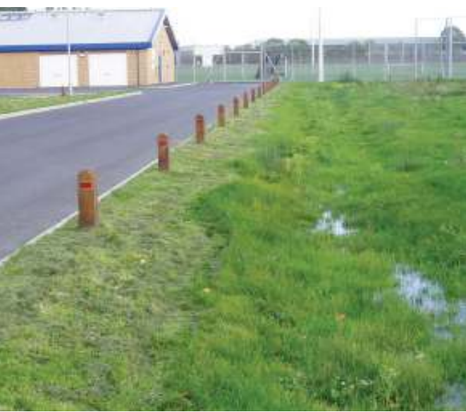
Pershore High School, Worcestershire. Low risk access road with 1.2m wide filter strip source control and conveyance swale.
