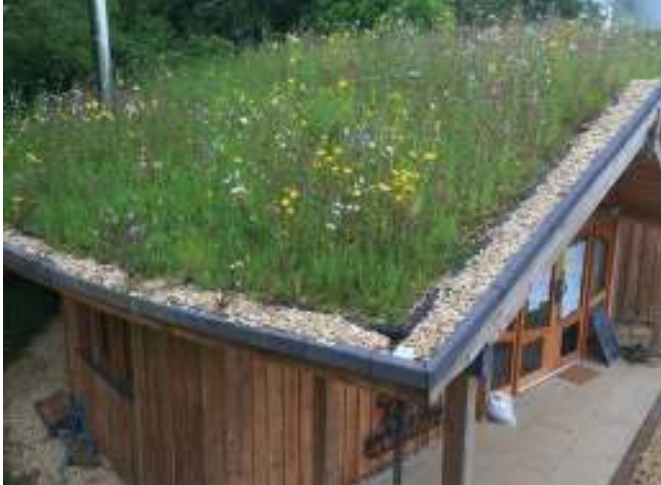
Ruskin Mill Horsely, Glos. Greenroof with gravel edge and rainchain.
