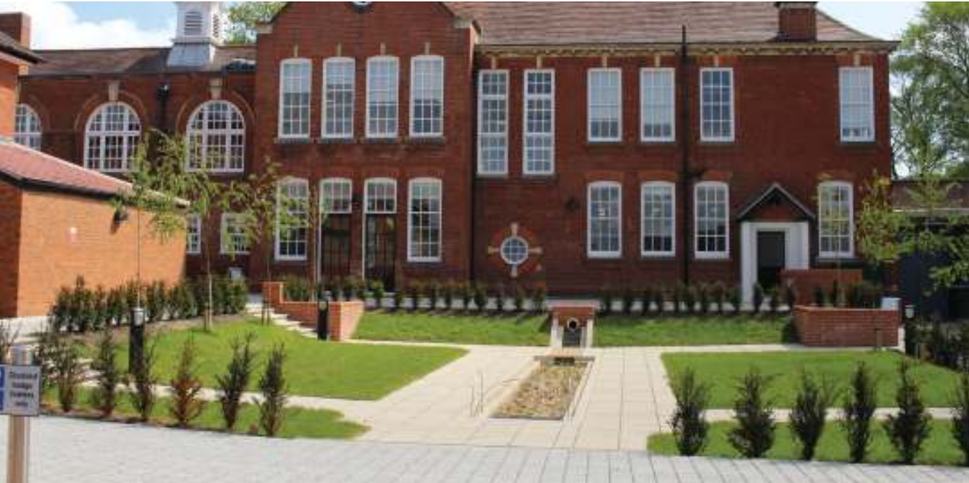
Bromsgrove Civic Centre re-development. Permeable block and slab paving with a central grass detention basin provide a fully integrated infiltrating SuDS scheme.
