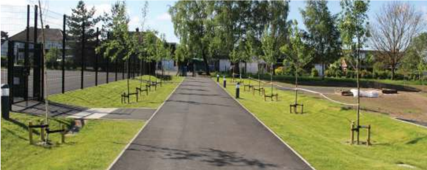
Linear swales alongside an entrance path at this infiltration SuDS project, Burlish Primary School.
