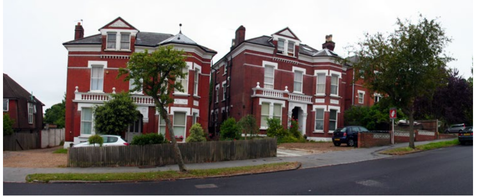
2-4 Hermitage Road (locally listed)
