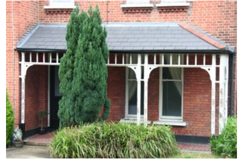
Well-preserved open porch
