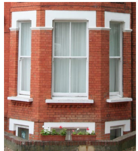
Original timber sash windows with lintel detailing above each window
