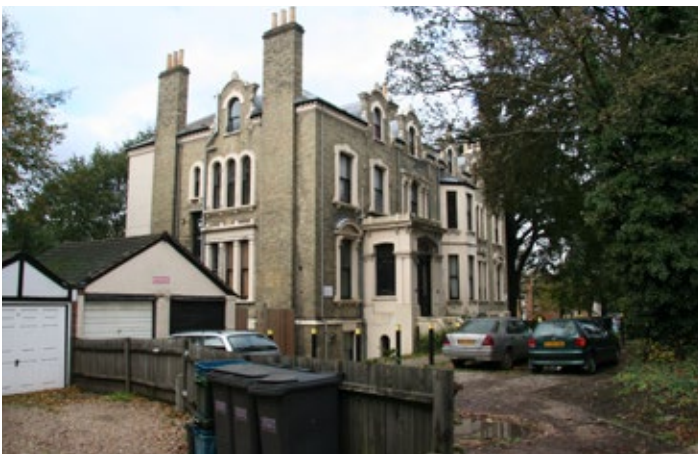
Side elevation of Cintra House
