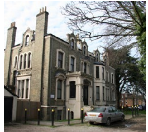
Cintra House, 9-11 Beulah Hill, locally listed
