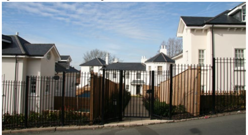
Numbers 2-4 Grange Hill (Gayfere), showing the restored Georgian buildings set back from the street behind high railings that are out of keeping with the character of the street
