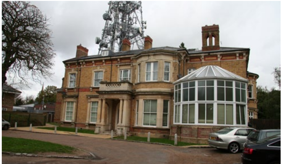
Beaulieu Heights Mansion. The NTL television mast in the background has a detrimental visual impact
