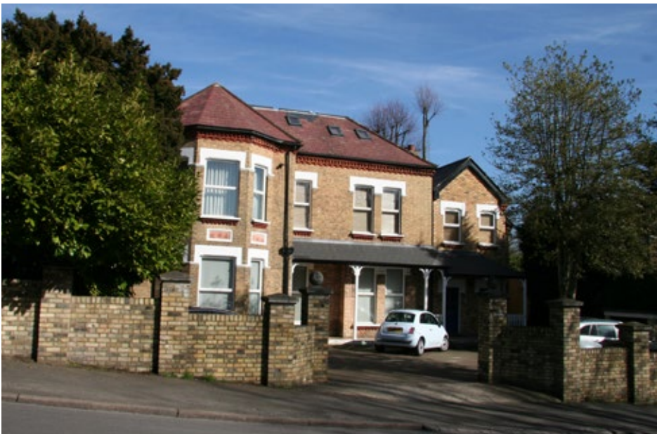
An example of a two-storey side extension to the right hand side of a building on Sylvan Hill. This extension would have been less visually intrusive if it had been set back from the front building line and had been of a smaller scale to preserve spacing between buildings
