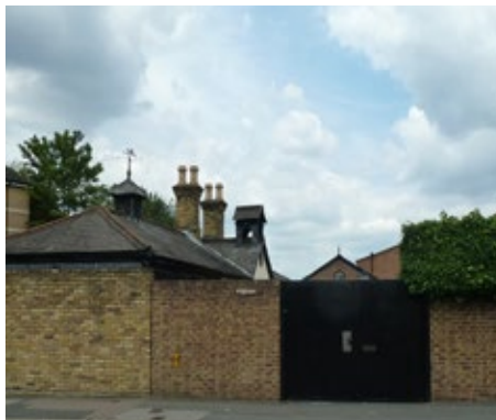
The roofscape of The Chimes, Upper Beulah Hill
