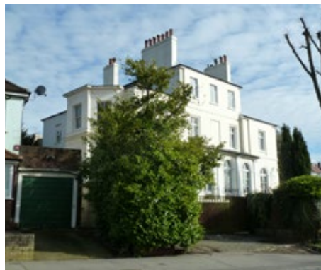
10 Grange Hill, late Georgian mansion now divided into flats
