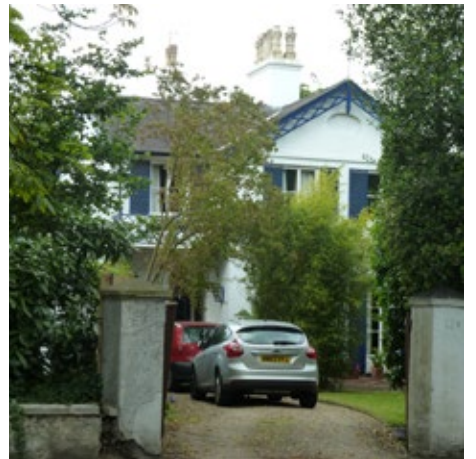
Beulah Villa 124 Church Road, Grade II listed
