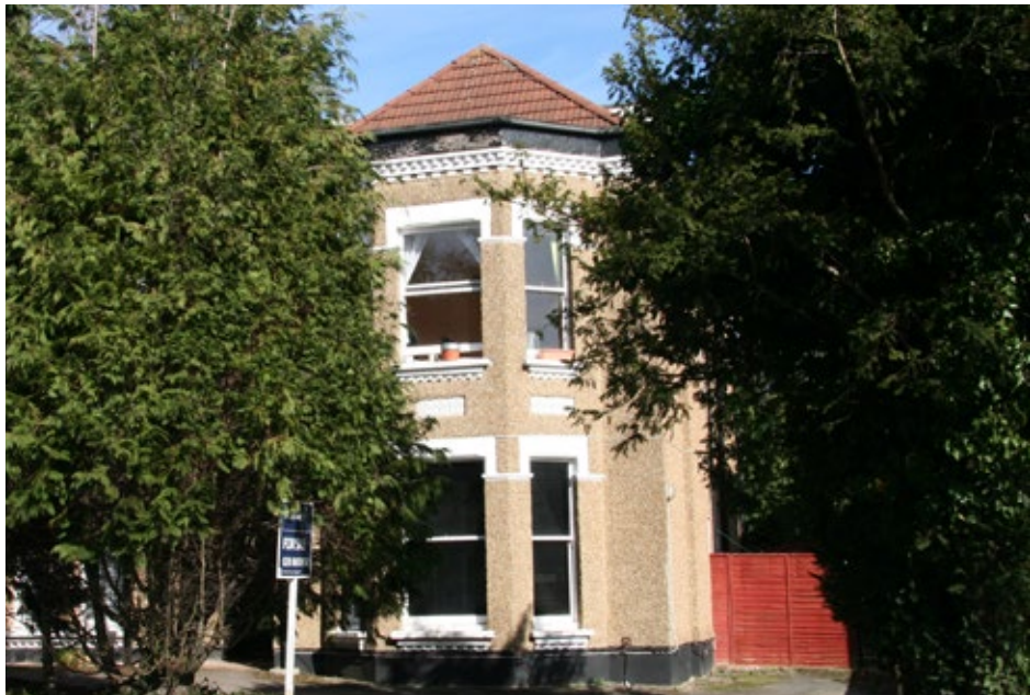
Pebbledash render over brickwork
