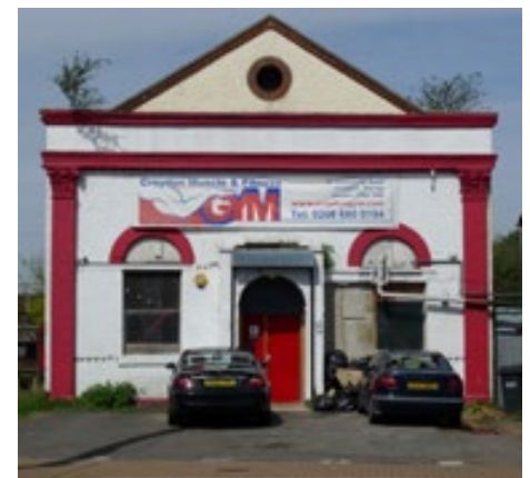
Locally Listed former Mission Chapel, Tamworth Road
