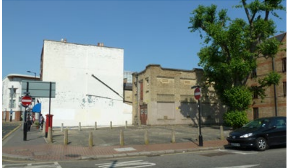
Open space in front of the substation at the corner of Church Road and Church Street
