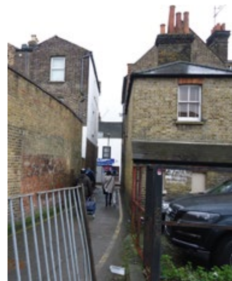
The pedestrian link from Church Street through to Drummond Road is in need of improvement
