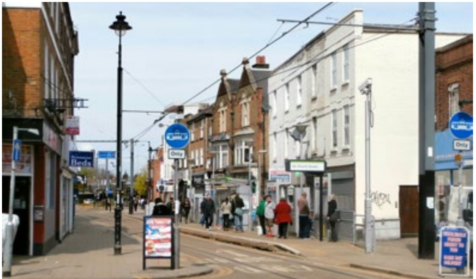
Numbers 82-98 Church Street, with the tram stop in front - this part of the street is cluttered due to the railings, signage and CCTV camera
