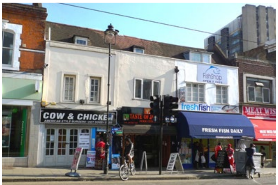
Distinctive historic pitched roofscape, set behind a parapet, at 21-25 Church Street
