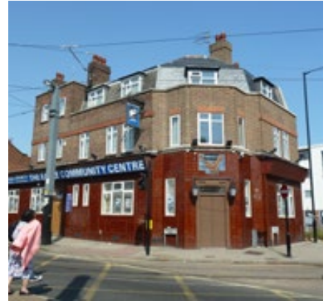
Former Eagle Public House
