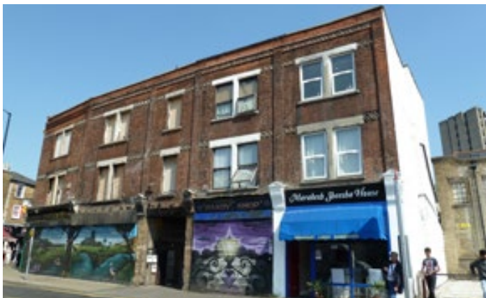
105-109b Church Street, facing Reeves Corner, which suffered fire damage during the 2011 Civil Disturbances
