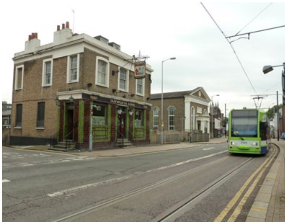
Tamworth Road streetscape, with the locally listed Tamworth Arms and Baptist Chapel (see pictures on p. 29)
