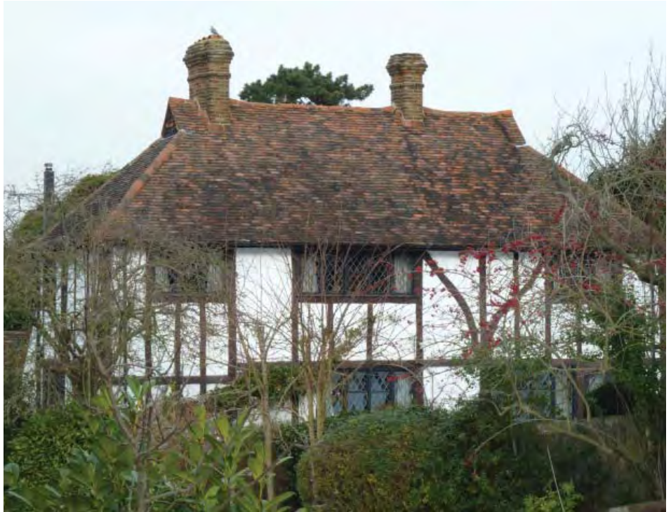
One of the Chapman Houses in the Croham Manor Road Conservation Area
