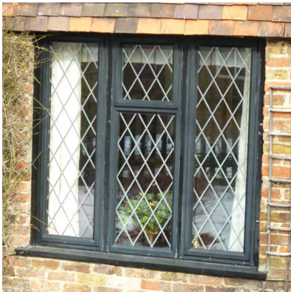
Sympathetic window replacement
