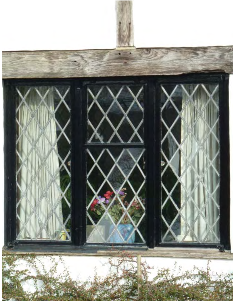
A timber framed leaded window, an architectural feature characteristic of the Croham Manor Road Conservation Area
