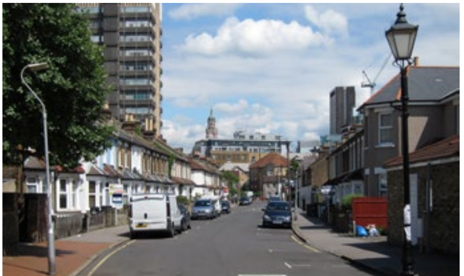
Howley Road has terraces with consistent building lines and shallow front gardens
