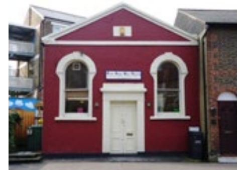
Former Wesleyan Chapel, locally listed, 26 Church Road
