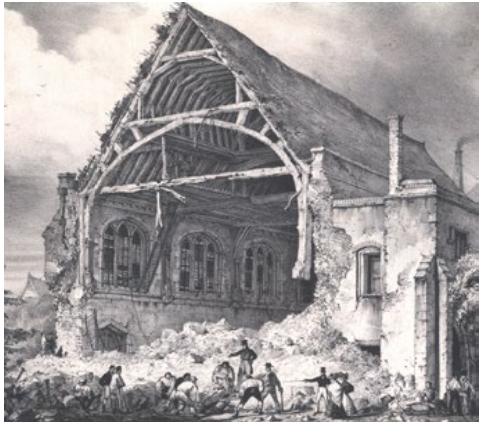
Engraving showing collapsed east wall of Great Hall at Croydon Palace, 1830
