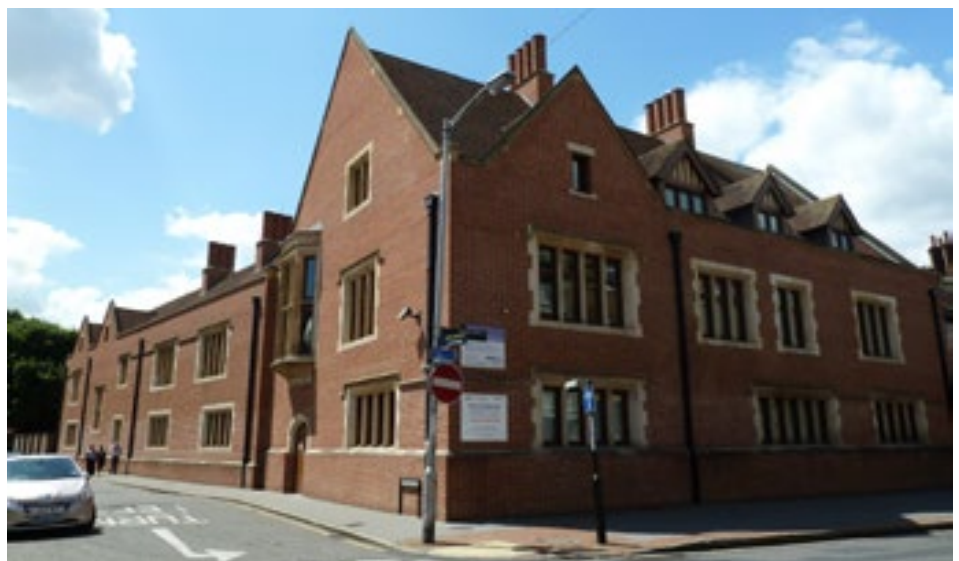
The Old Palace Preparatory School building, built in 2001 on the corner of Church Road and Old Palace Road, is a high quality modern development of a contemporary design by Porphyrios Architects in a Tudor style. Built in red brick with crisp limestone dressings, it is. It respects and complements its important historic context and is a valuable addition to the Old Town area.
