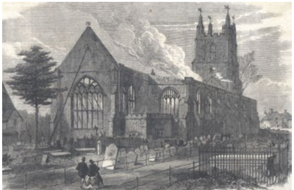
Etching showing St John's Church almost destroyed by fire in 1867
