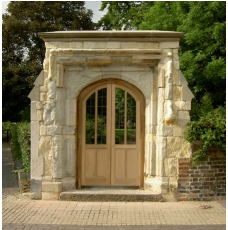
The Tudor Arch (St John's Gateway), a scheduled monument, photographed soon after repairs carried out in 2006
