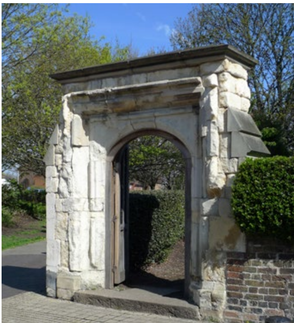
The Tudor Arch (St John's Gateway) Scheduled Monument, located at the west end of Howley Road at the entrance to the St John's Memorial Garden - it is at present the only scheduled monument in Croydon's town centre
