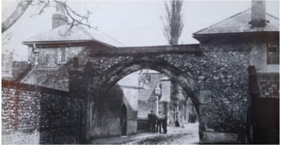
Old Palace Road c.1880 - the Old Palace Archway, demolished 1880s, was located just to the south of the present junction with Church Road (source: Croydon Past , John Gent)
