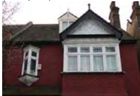
Plasterwork detailing at number 170
