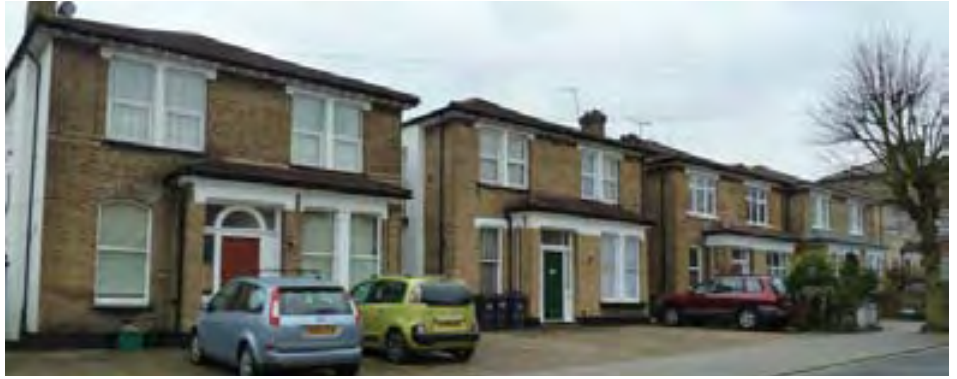
Loss of front gardens to properties on Clyde Road, leaving a stark and harsh appearance and negative impact on the streetscene
