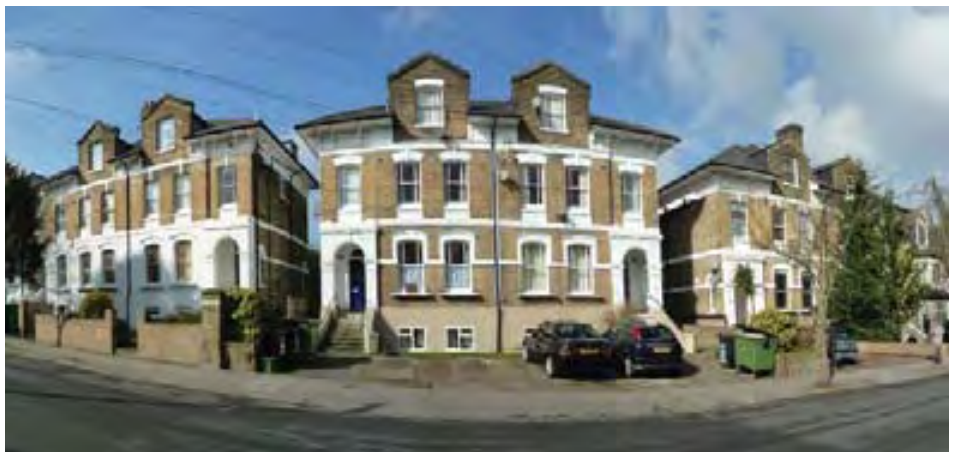
Typical sequence of three storey pairs of semis on Outram Road
