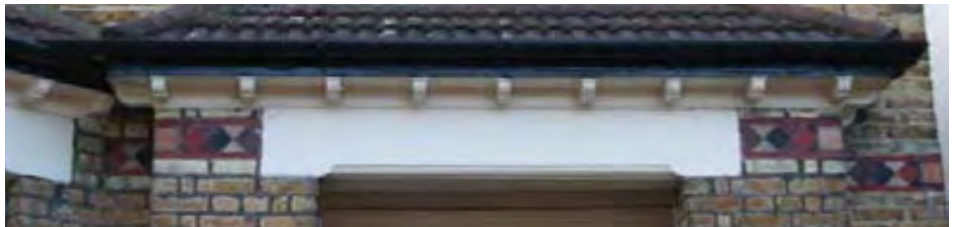
Decorative window framing at 87 Elgin Road
