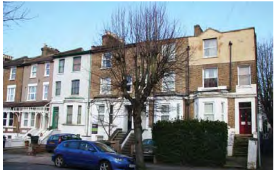
Examples of inappropriate cladding and render that has harmed the unity of this Victorian terrace
