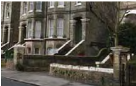
Low walling boundary treatment with brick piers topped with stone coping
