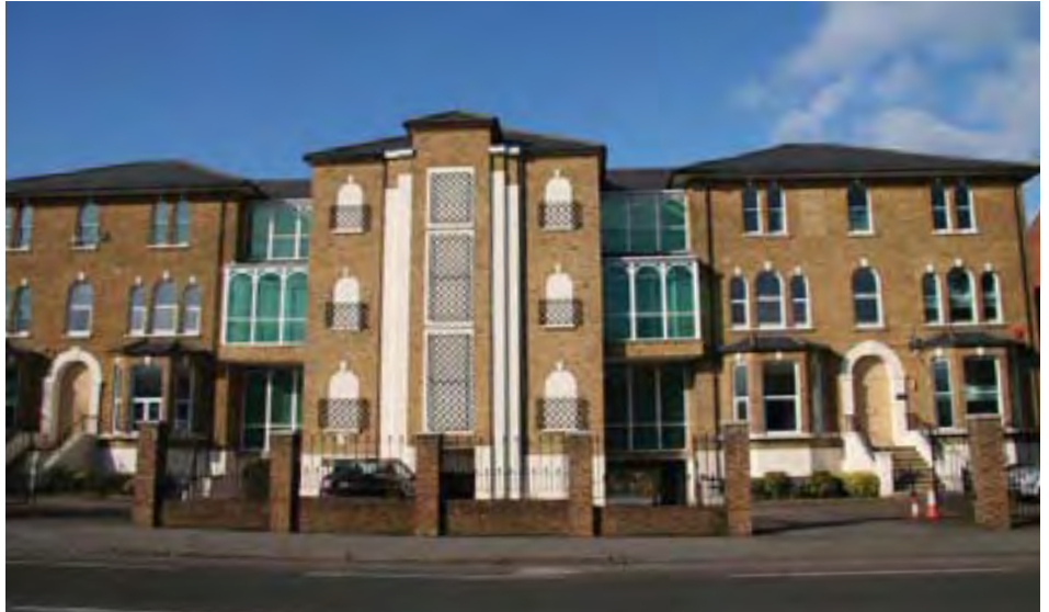
Pairs of semi-detached buildings that have been conjoined.
