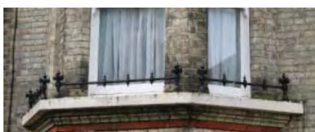
Architectural detailing of London brick elevations
