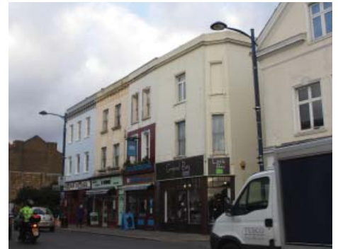
Three storey terraced buildings on Westow Street
