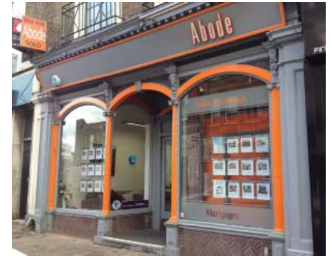
Historic shopfront at 80 Westow Hill
