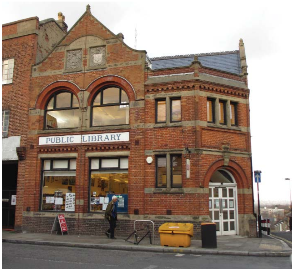
The historic Upper Norwood Library makes an important contribution to the streetscape of Westow Hill, within the setting of the Upper Norwood Triangle Conservation Area
