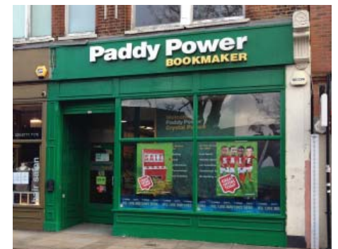
Traditionally designed modern shopfront at 47-49 Westow Street
