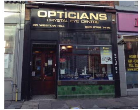
Historic shopfront at 20 Westow Hill
