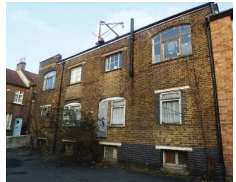
Haynes Lane workshops, with 10-11 Haynes Lane visible behind
