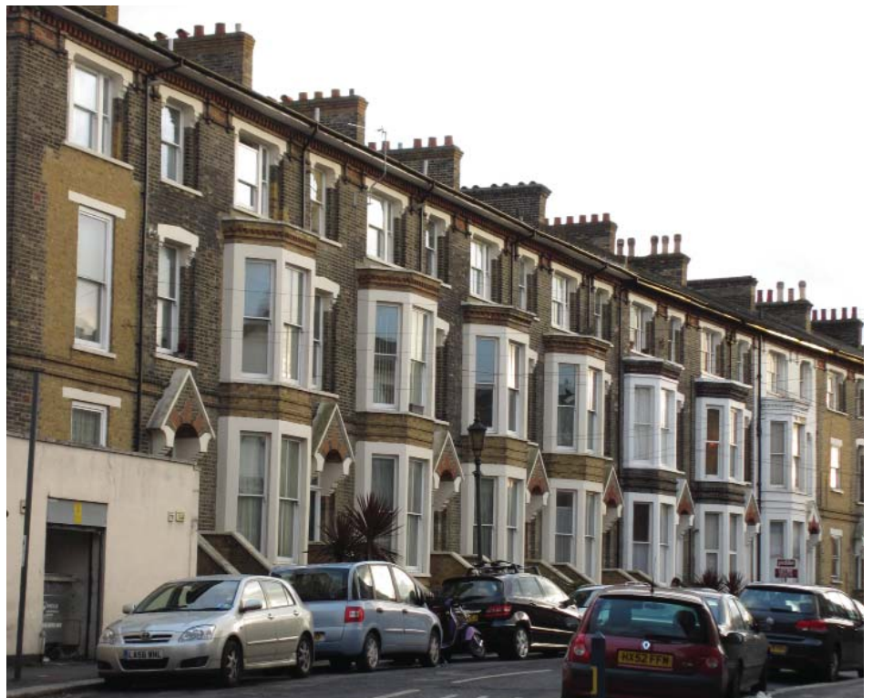
Terraced houses on the east side of St Aubyn's Road
