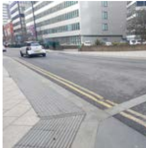
Far left: New Street, Brighton. Gully and tactile paving create a "safe zone"
