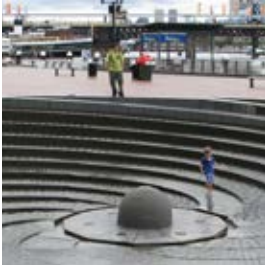
The water feature in Darling Harbour, Sydney changes in levels, creating an HVM barrier
