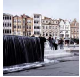
The water feature on Market Square in Nottingham, combines vertical elements and changes in levels, creating an HVM barrier
