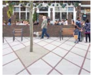
Bespoke pavers in South End to be replaced by standard ones at the end of their life
