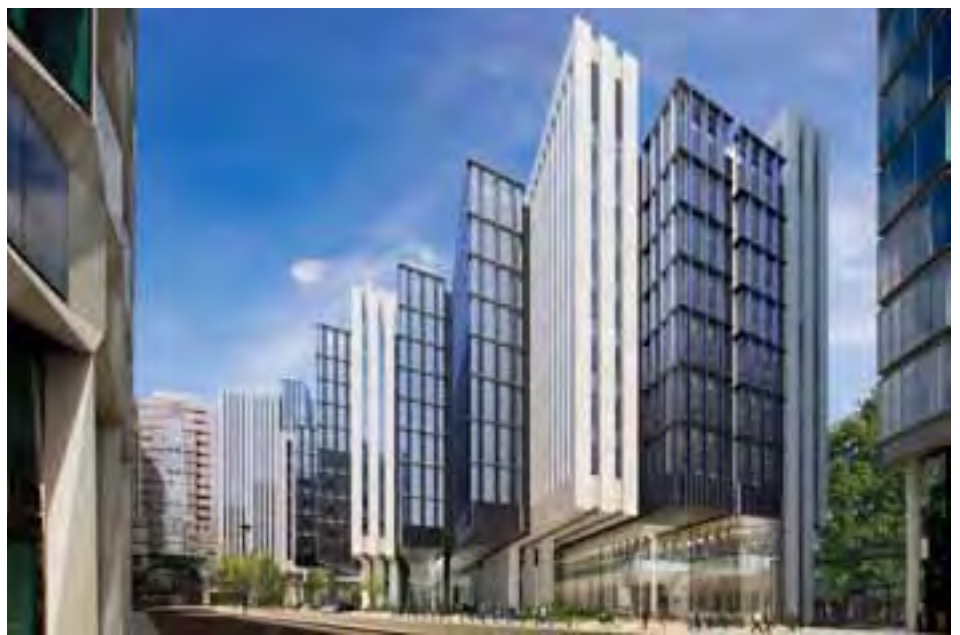
Breaking the massing of the block into individual elements can help to make the most of the linear site.
