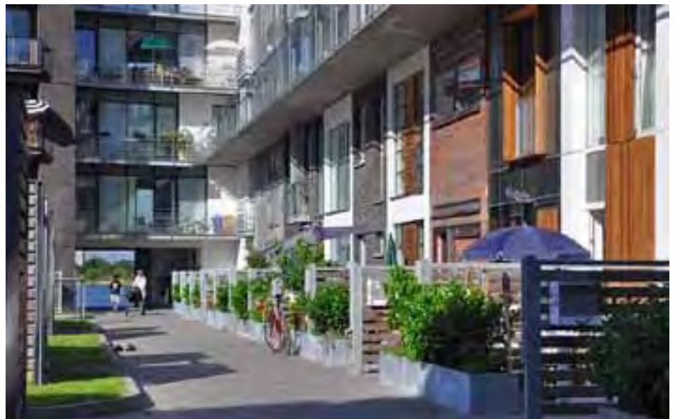
Development blocks visually broken up into smaller elements through the use of materials to better relate to a human scale
