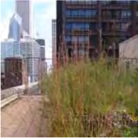
Biodiversity green roof
