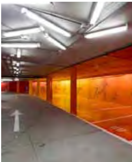
Brighter, safer car park to improve quality of access via subway
