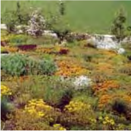
Biodiversity green roof
