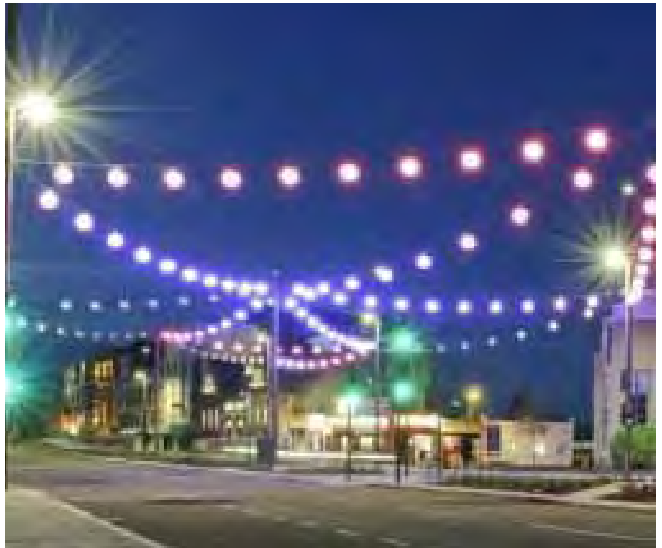
Use of catenary lighting
