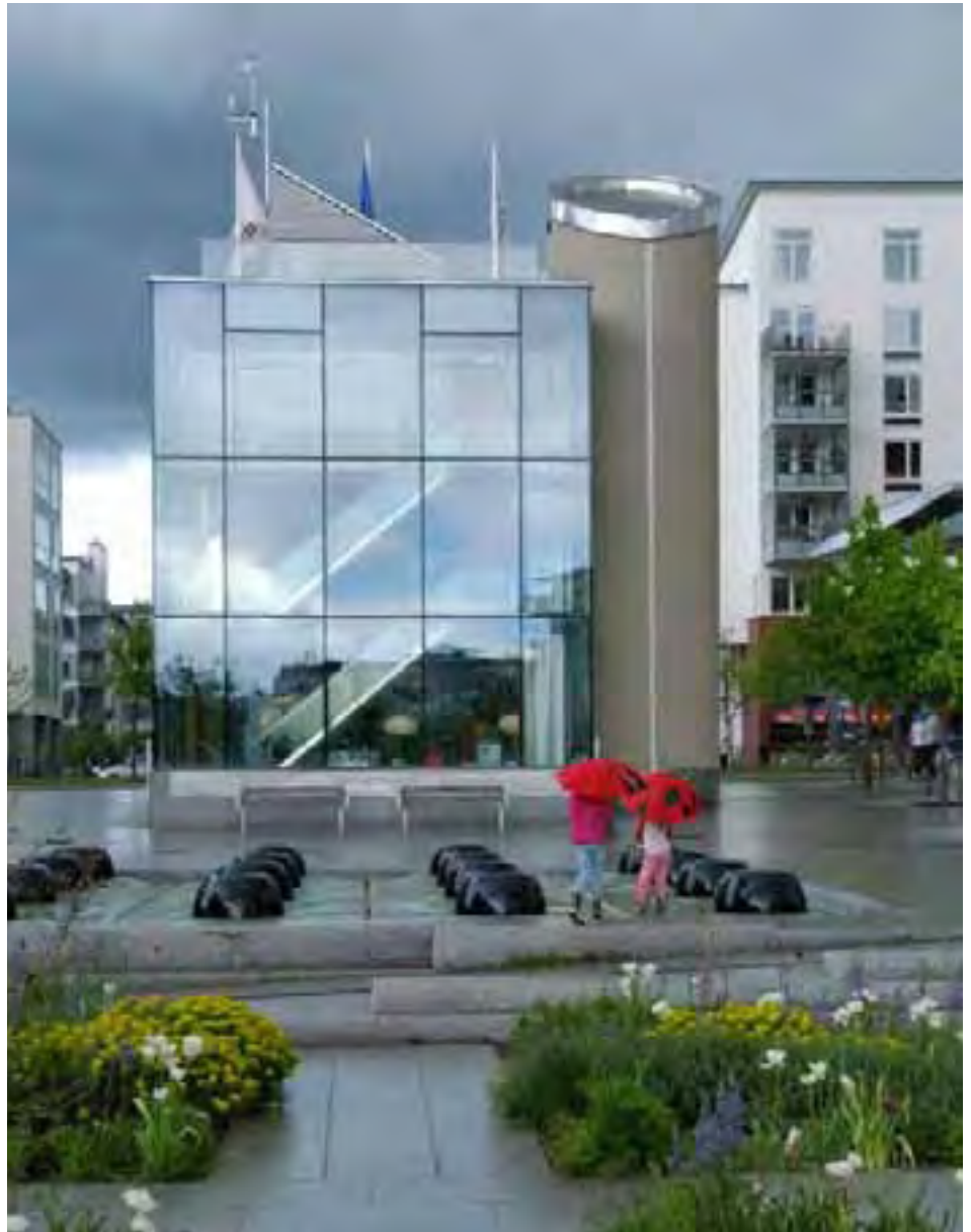
Long term: there may be opportunities to turn into a site wide energy centre with key elements on display for public promotion / education.
