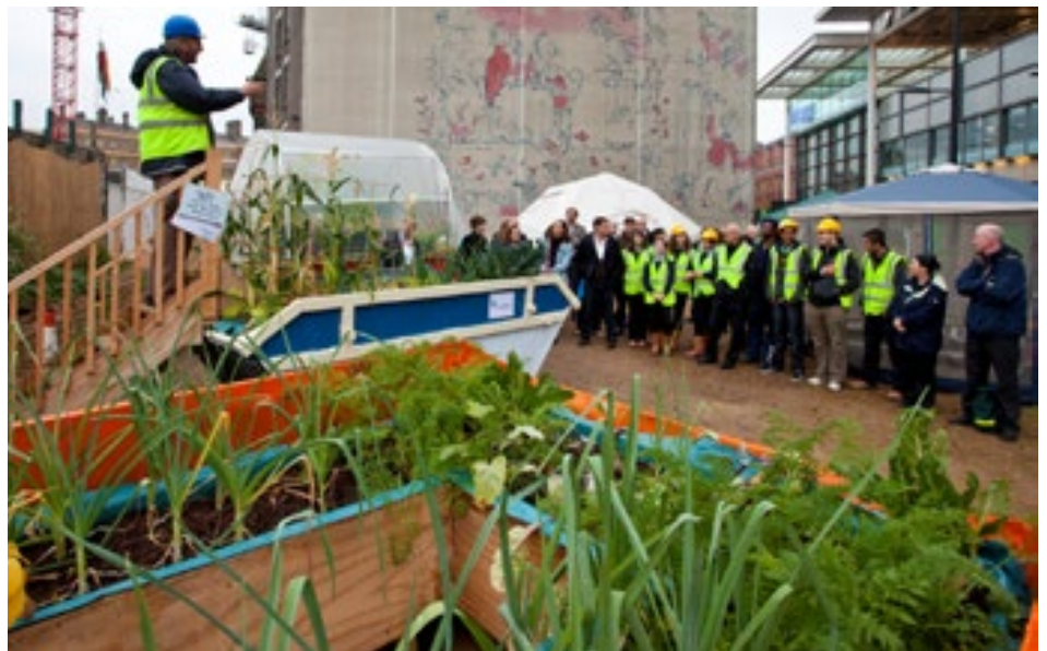
Temporary skip gardens during construction at Kings Cross. This project is ongoing and now has a pop-up cafe
