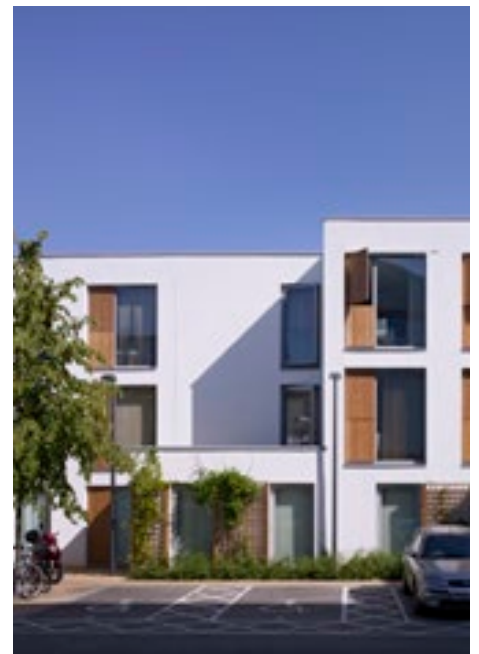
Car parking, bike parking and planting within developments, Arsenal, London - Allies and Morrison
