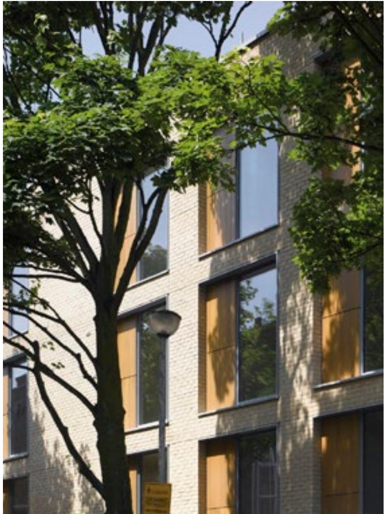
High quality facade detailing and materials. Greenery makes an important contribution towards the attractiveness of these spaces. Highbury Square, London - Allies and Morrison
