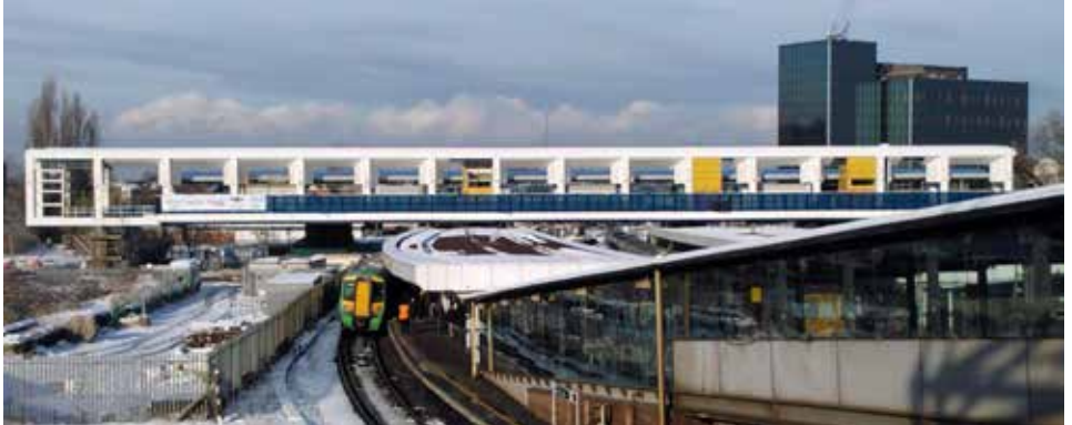
THE CONSTRUCTION OF EAST CROYDON BRIDGE
