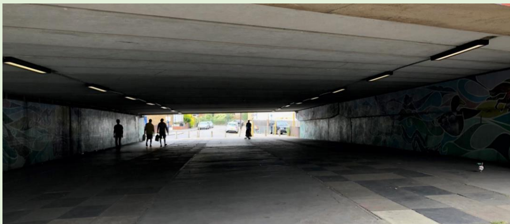
Pedestrian underpass at Reeves Corner
